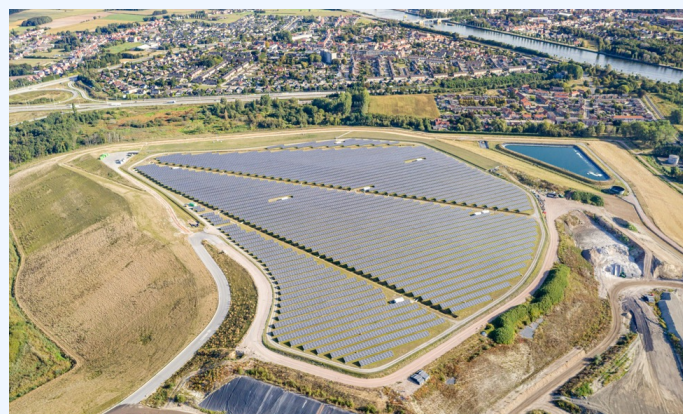
Fig 22. Terranova solar park 123
